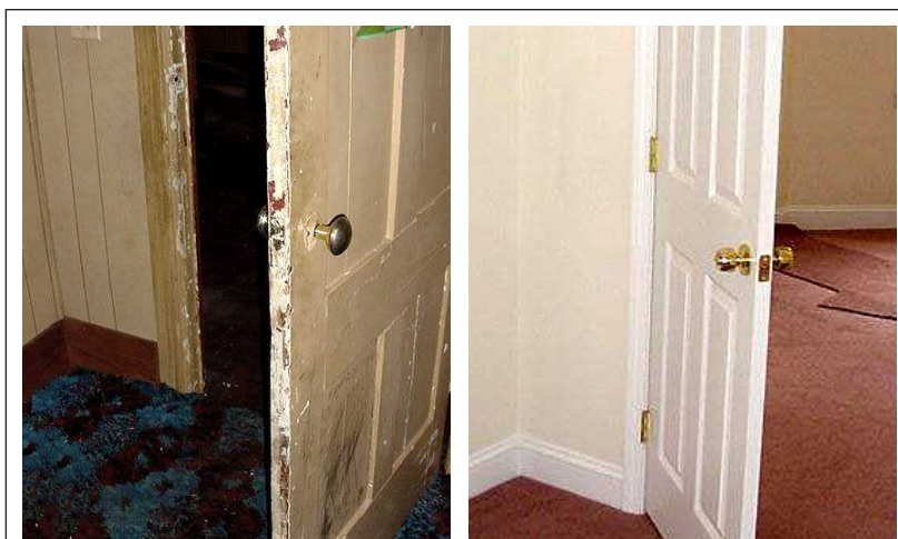
FIGURE 12.4 Pre-and post-abatement interior doors.
