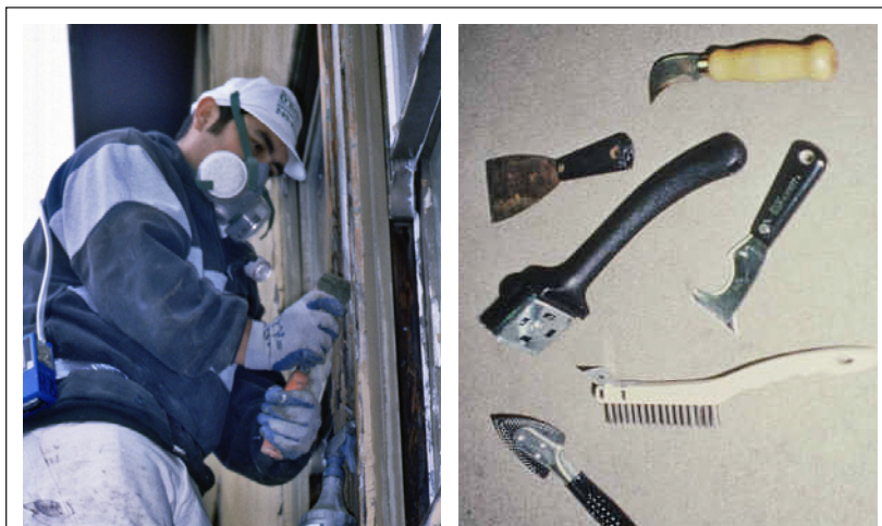
FIGURE 12.16 Wet scraping (left) FIGURE 12.17 Scraping tools (right).
