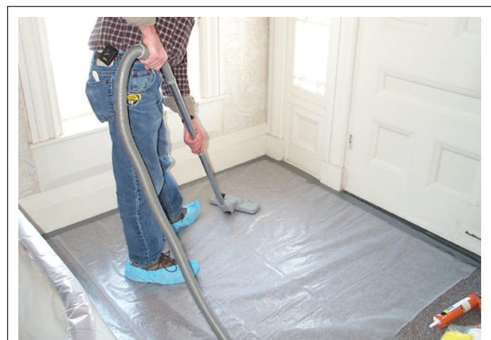
FIGURE 4.4 HEPA vacuuming is an important step in the specialized cleaning process.
