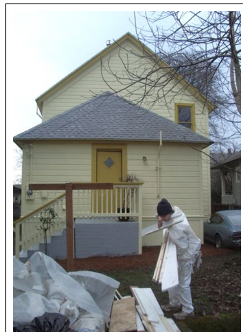
FIGURE 10.1 Separate waste into categories during work.
